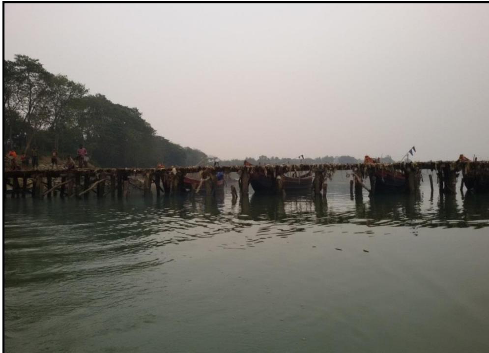
WOODEN BRIDGE PATNA CHAINAGE 258 KM
