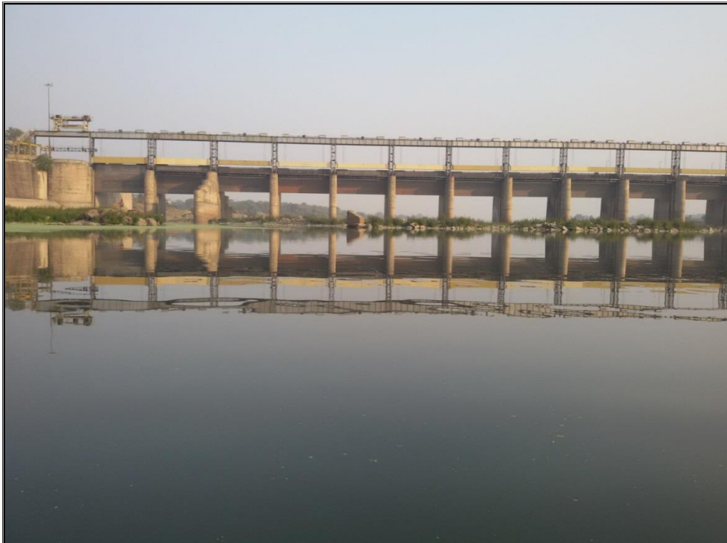
DIGRI BARRAGE AT CHAINAGE 75 KM
