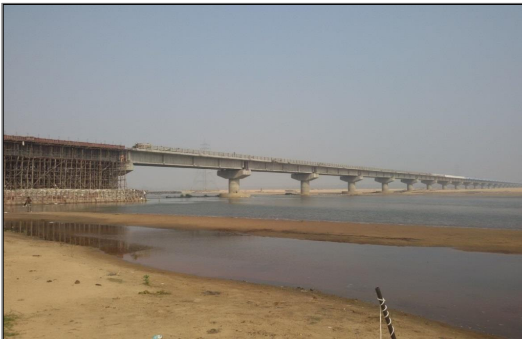
MAJOR BRIDGE UNDER CONSTRUCTION AT BHASRA GHAT CHAINAGE 217 KM
