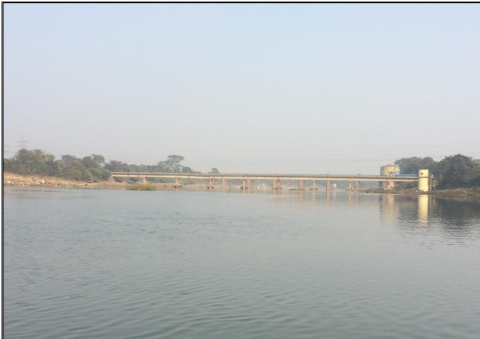
BASRA GHAT BRIDGE AT CHAINAGE 216.6 KM
