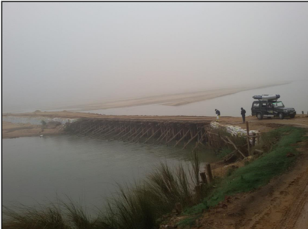
WOODEN BRIDGE AT CHAINAGE-243 KM SONAKANIA
