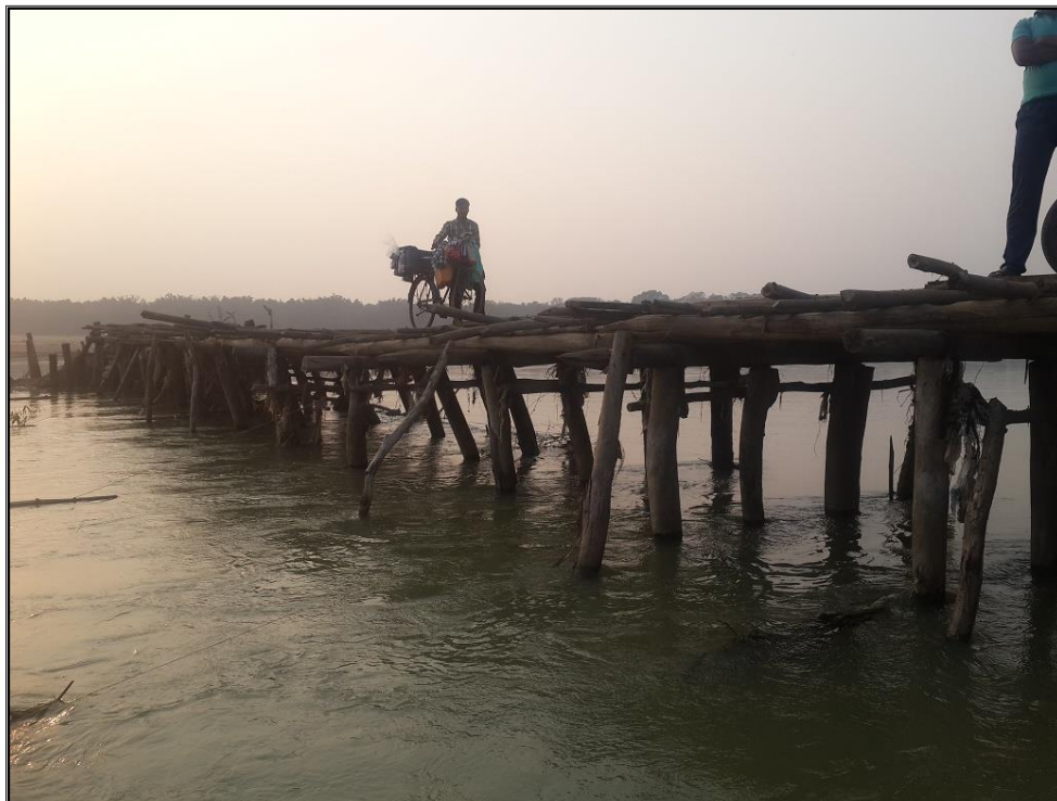
WOODEN BRIDGE PHULBONI CHAINAGE 208 KM
