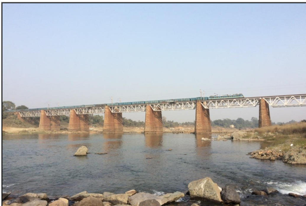
MANIKUI RAILWAY BRIDGE CHAINAGE 12.5
