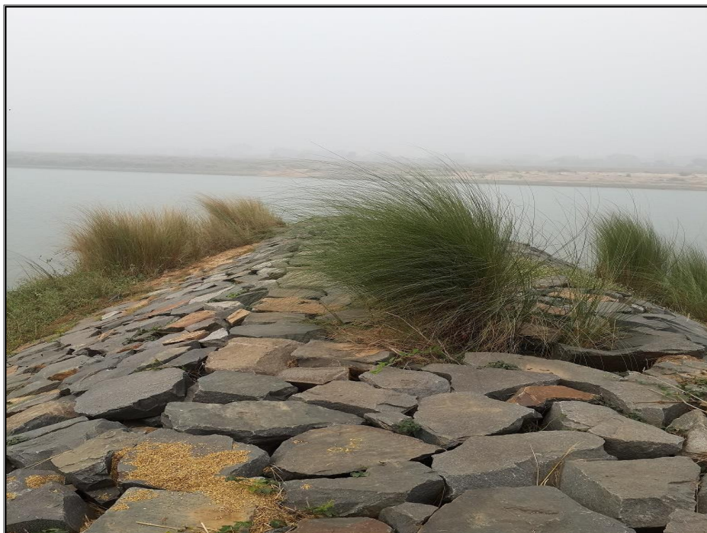
BREAKWATER BISHNUPER CHAINAGE 291 KM
