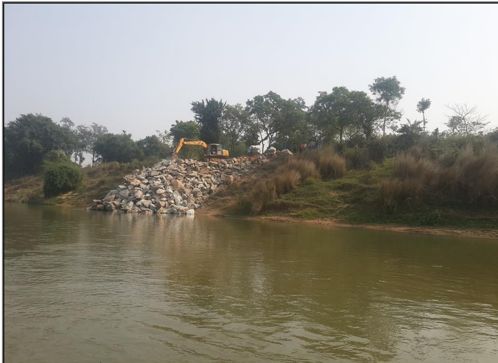
CONSTRUCTION OF BREAKWATER MAKRAMPUR CHAINAGE 246 KM
