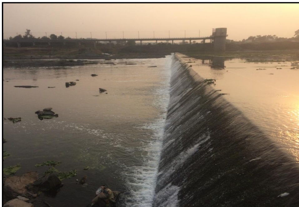
PURUBHAT DAM CHAINAGE 49 km
