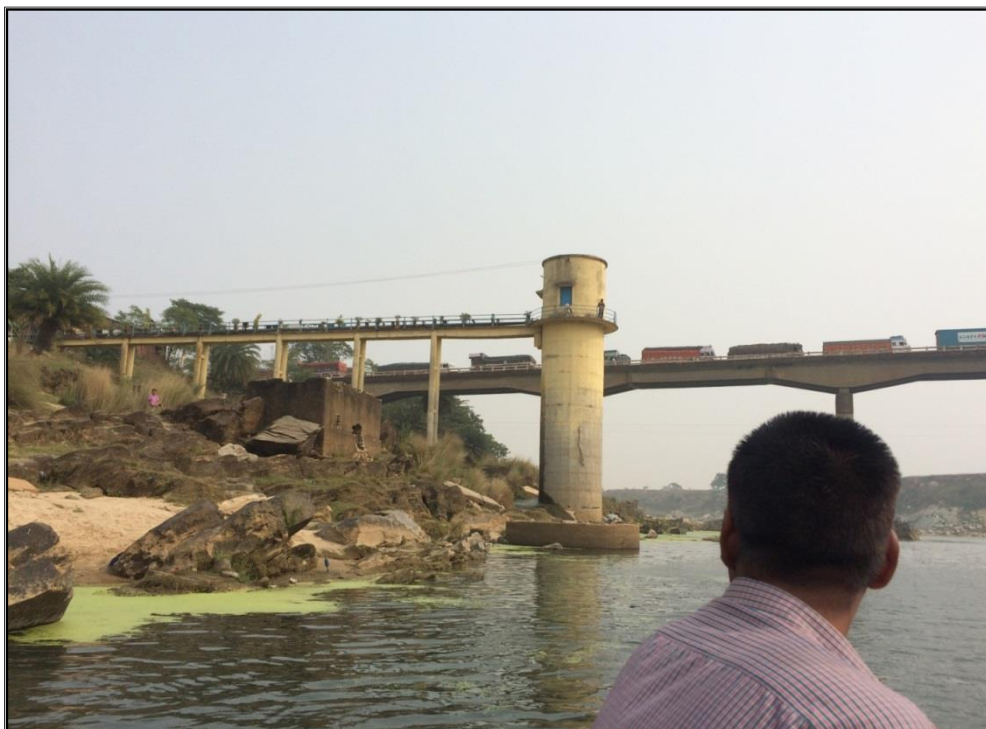
JAMSHOLA BRIDGE CHAINAGE 145 KM
