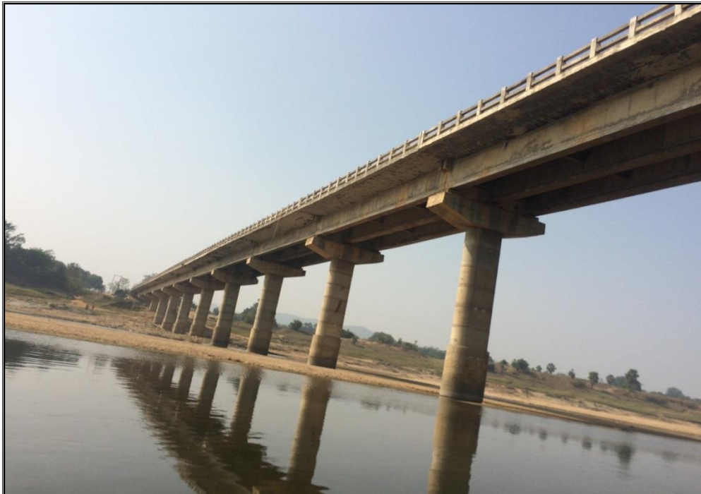
DEDANG BRIDGE AT CHAINAGE 101 km
