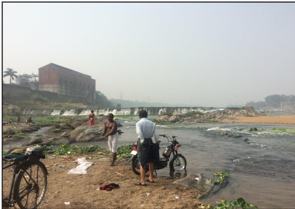
MANGO DAM CHAINAGE 34.5 km
