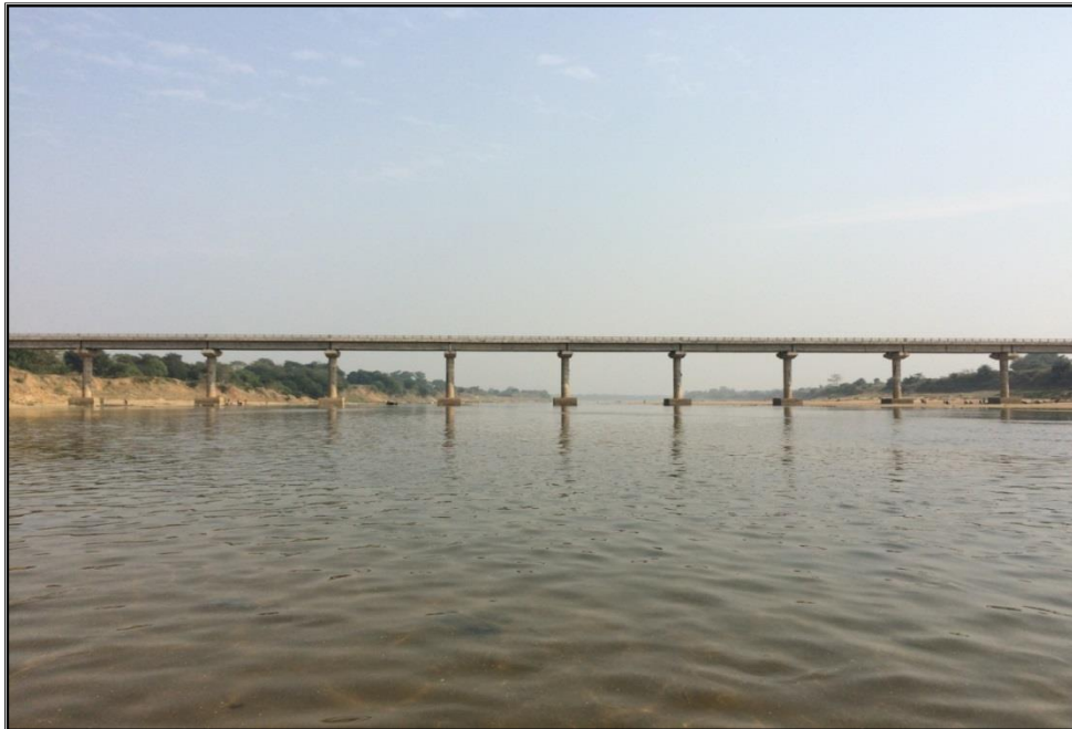
MAJOR ROAD BRIDGE BINDA CHAINAGE 107 KM
