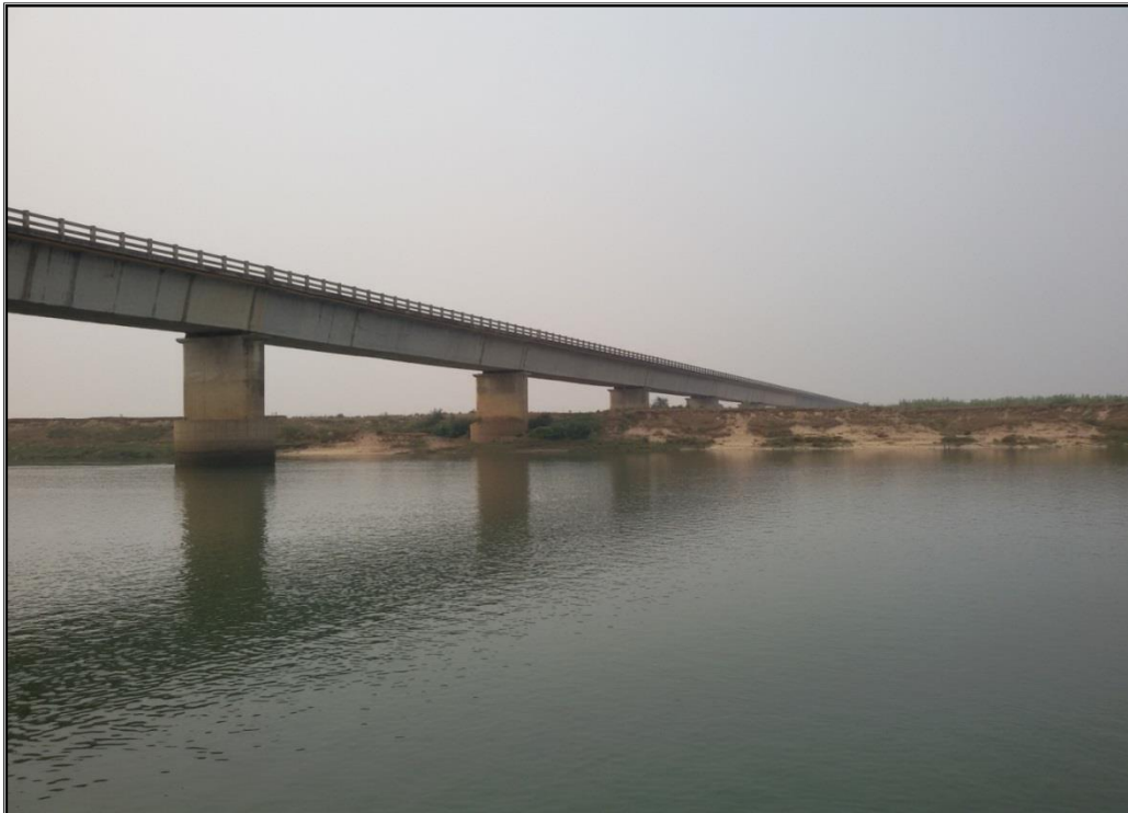
KATHAPAL MAJOR ROAD BRIDGE CHAINAGE 286 KM
