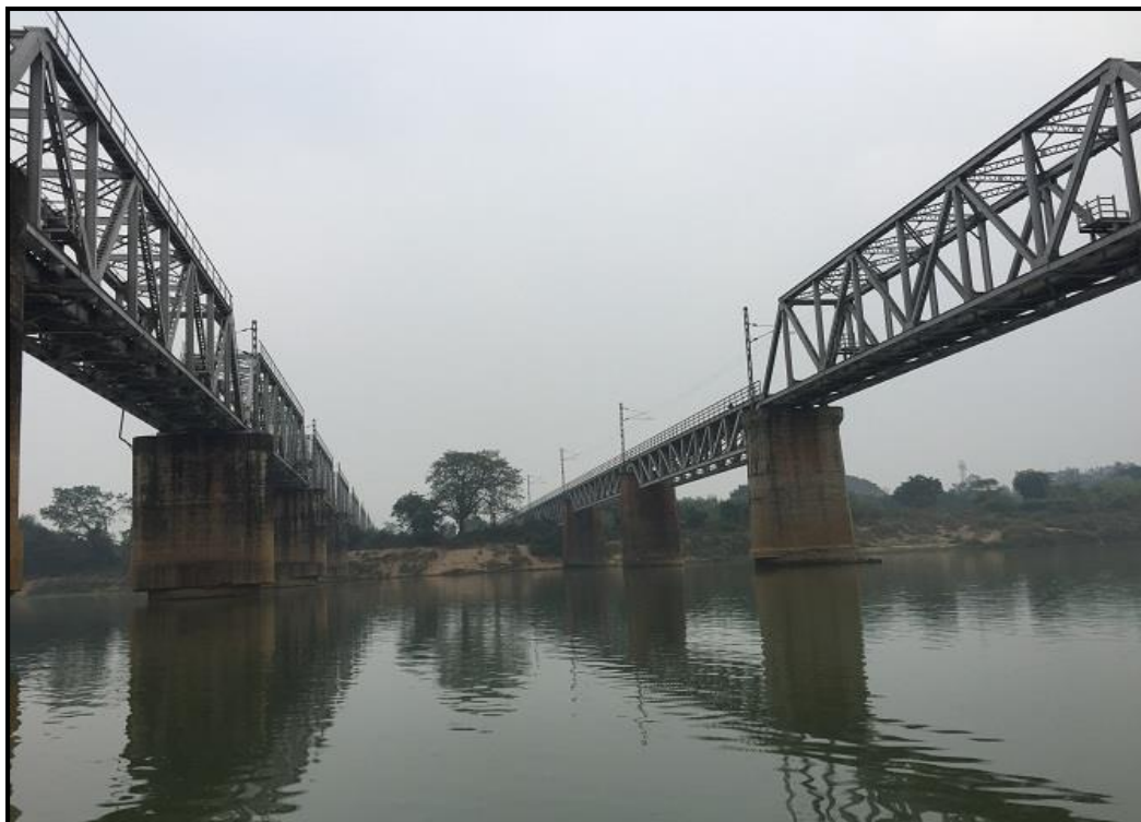
RAJGHAT RAIL BRIDGE CHAINAGE 262 KM
