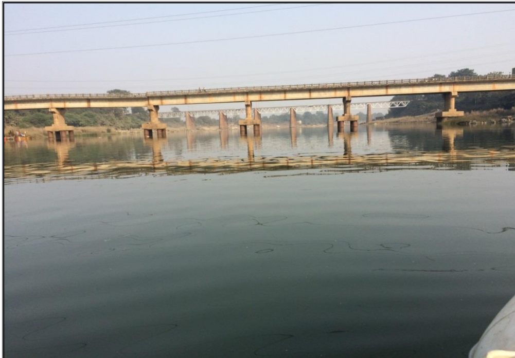
MANIKUI BRIDGE CHAINAGE 12 km
