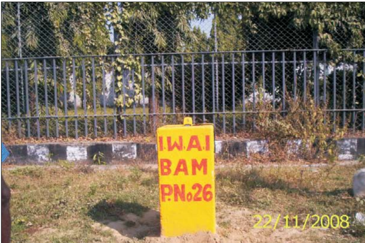
Survey Pillar constructed in National Waterway No.1 (Location: Mokama )
