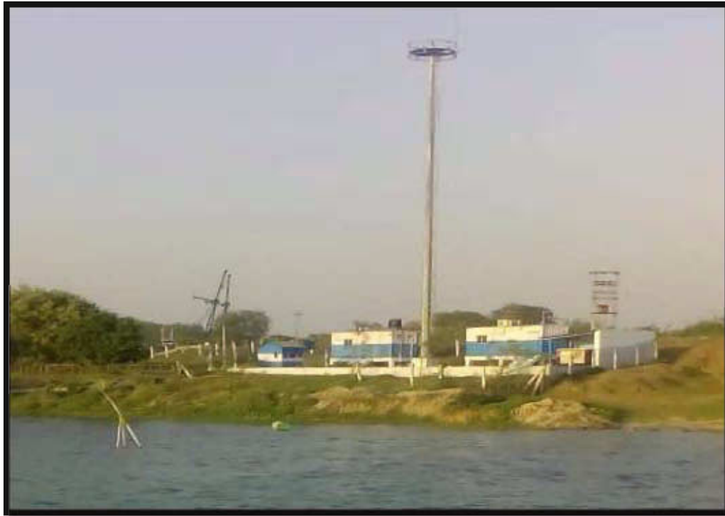
River View of Farakka RIS Control station
