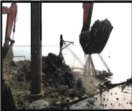
Removal of Hard Strata in progress on National Waterway-1
