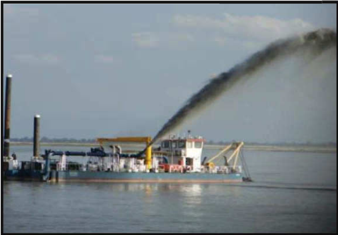
Dredging at Pandu by CSD Mandovi
