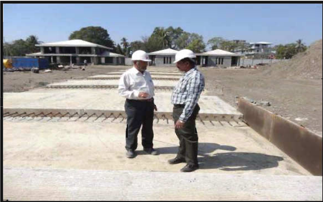
ROAD AND CIVIL WORKS UNDER CONSTRUCTION AT SITTWE, MYANMAR
