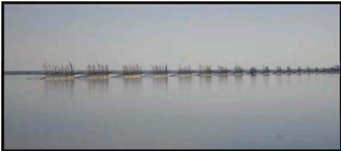
Bandal erected along National Waterway-1
