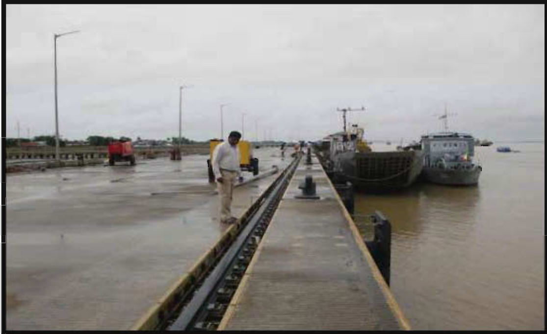
NEWLY CONSTRUCTED PORT JETTY AT SITTWE (NAVY VESSEL IS BERTHED)
