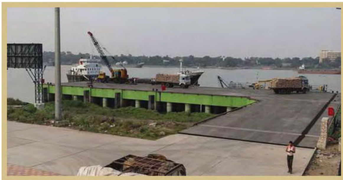
Permanent Terminal at G R Jetty-2 Kolkata
