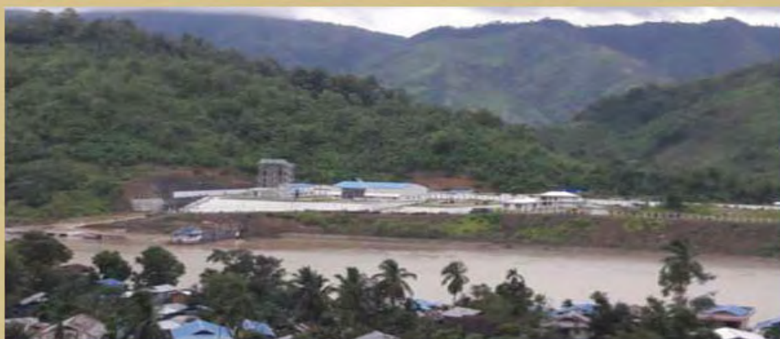
Construction of IWT Jetty at Paletwa
