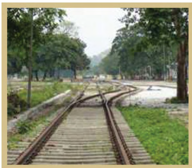
Road-Rail Linkage at Pandu Terminal
