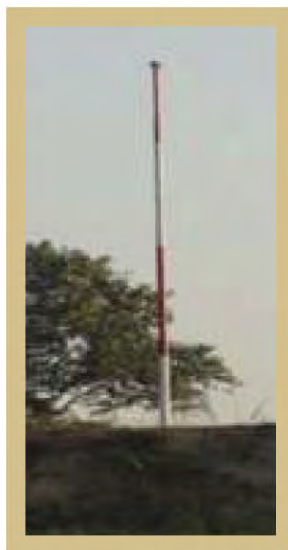
Light on Steel Pole
