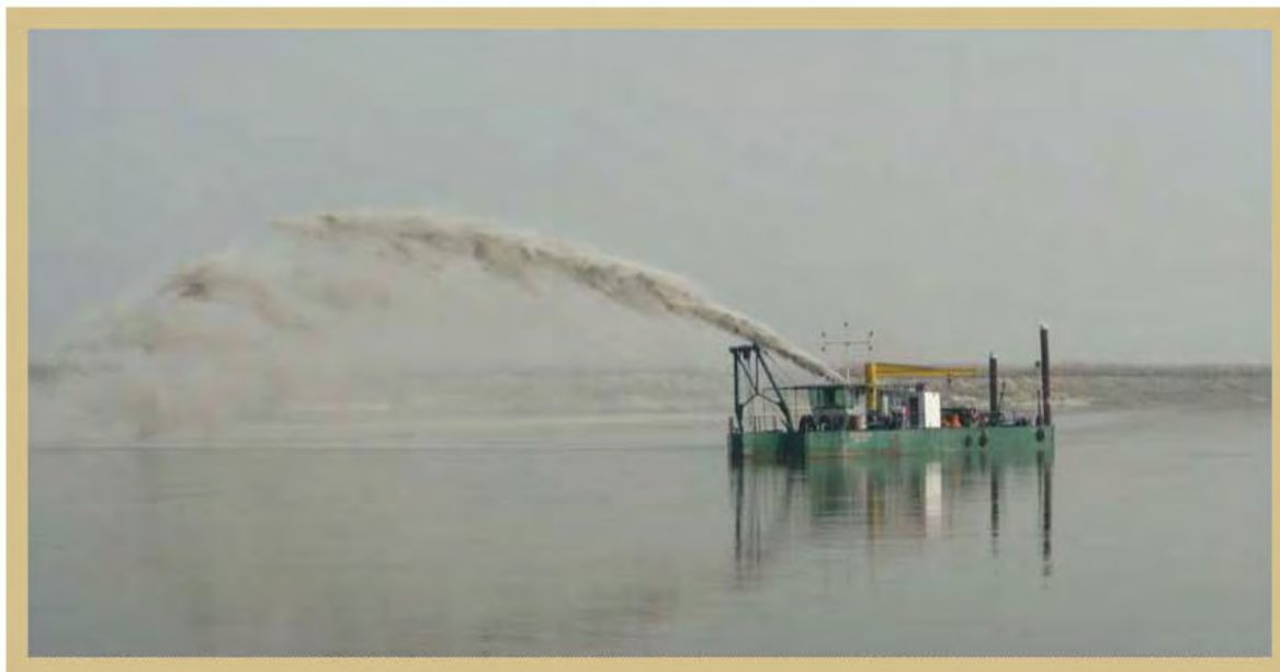
Dredging in progress on National Waterway-1
