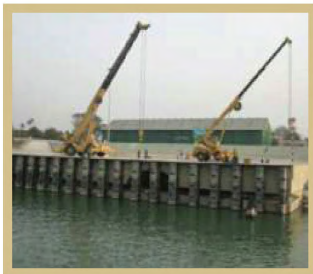
Terminal with cargo handling equipment on NW-2
