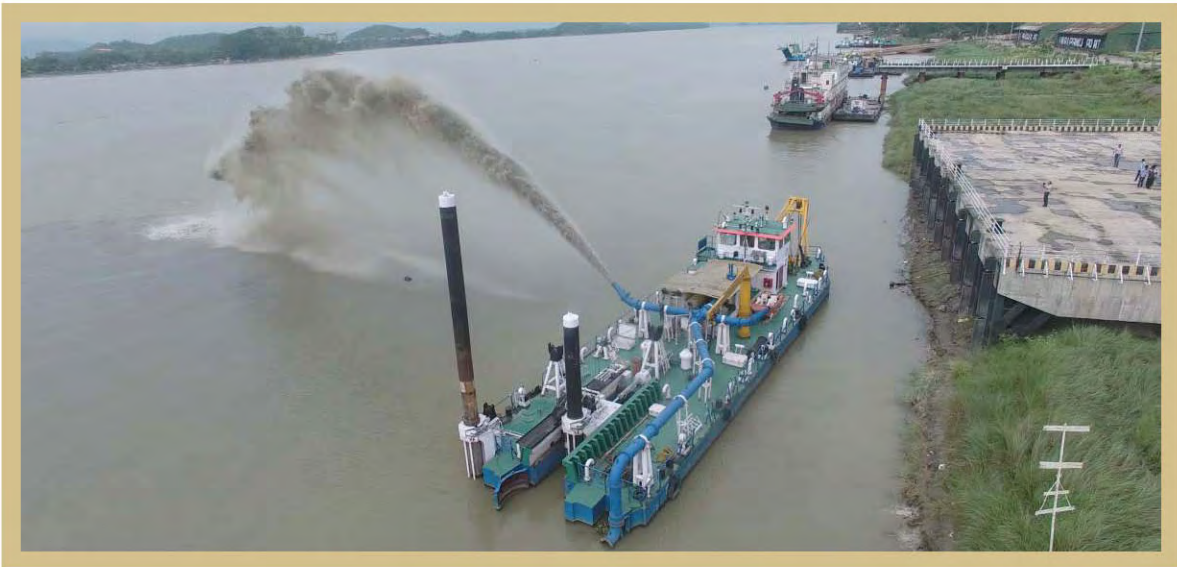
Dredging at Pandu by CSD Mandovi
