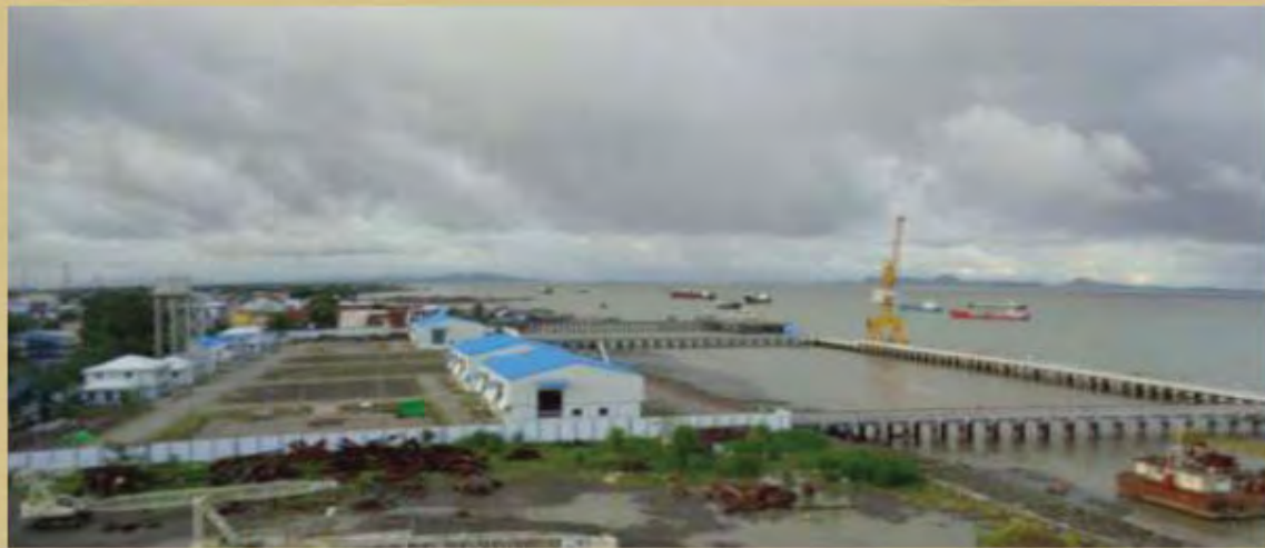
Construction of Port & backup facilities at Sittwe
