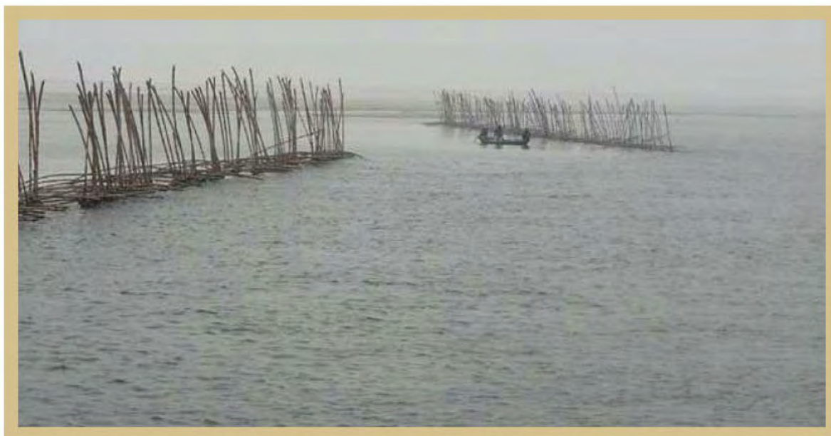
Bandal erected along National Waterway-1
