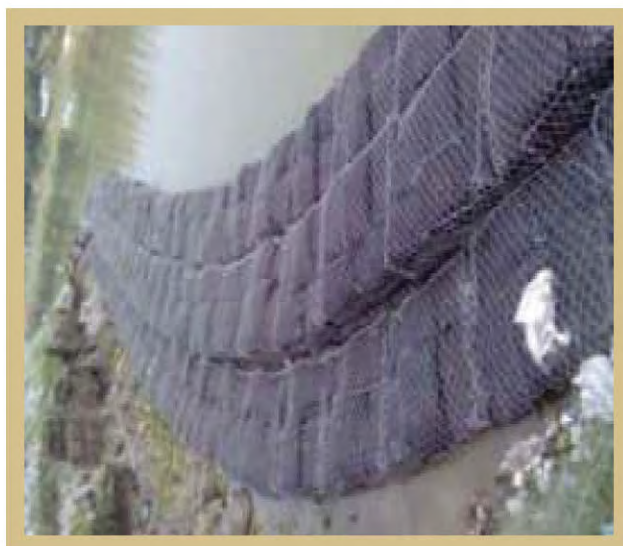
Bank Protection Works at Jogighopa
