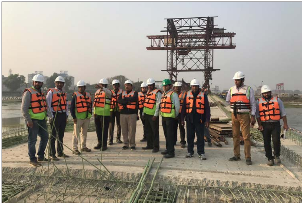
World Bank team visit to IWAI, MMT IWT Terminal at Haldia
