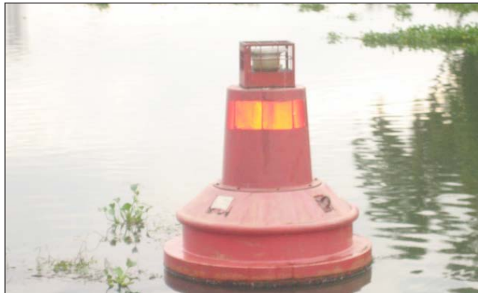
Solar Powered FRP Buoy installed in NW-3
