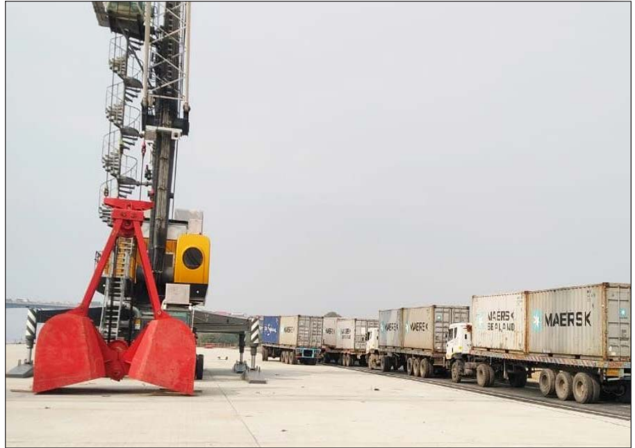
Figure 3- NW-1: Multimodal Terminal at Varanasi
