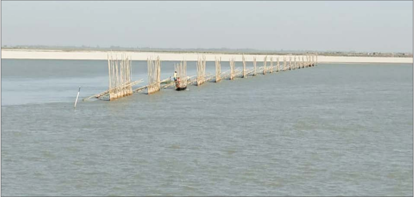
Bandal erected along National Waterway-1
