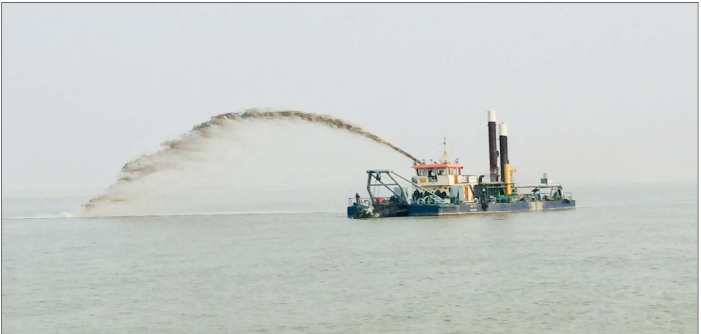
Dredging in progress on National Waterway-1
