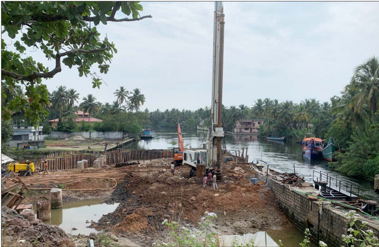
Piling work for Thrikkunnappuzha Lock construction is in progress
