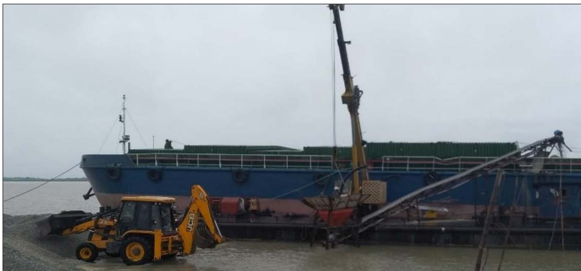
Figure 27- NW-2: Loading operations at Dhubri jetty
