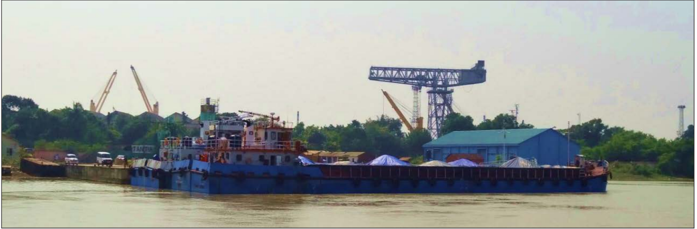
Permanent Terminal at G R Jetty-2 Kolkata
