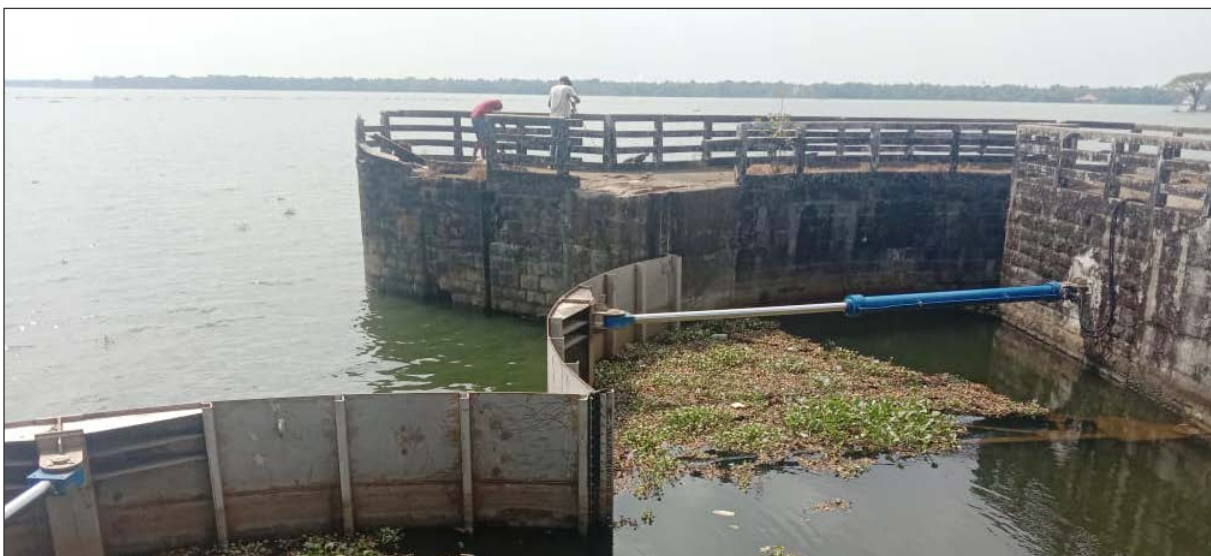
View of renovated Thanneermukkam 40' Lock
