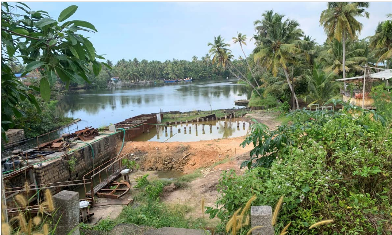
Piling work for Thrikkunnapuzha Lock construction is in progress
