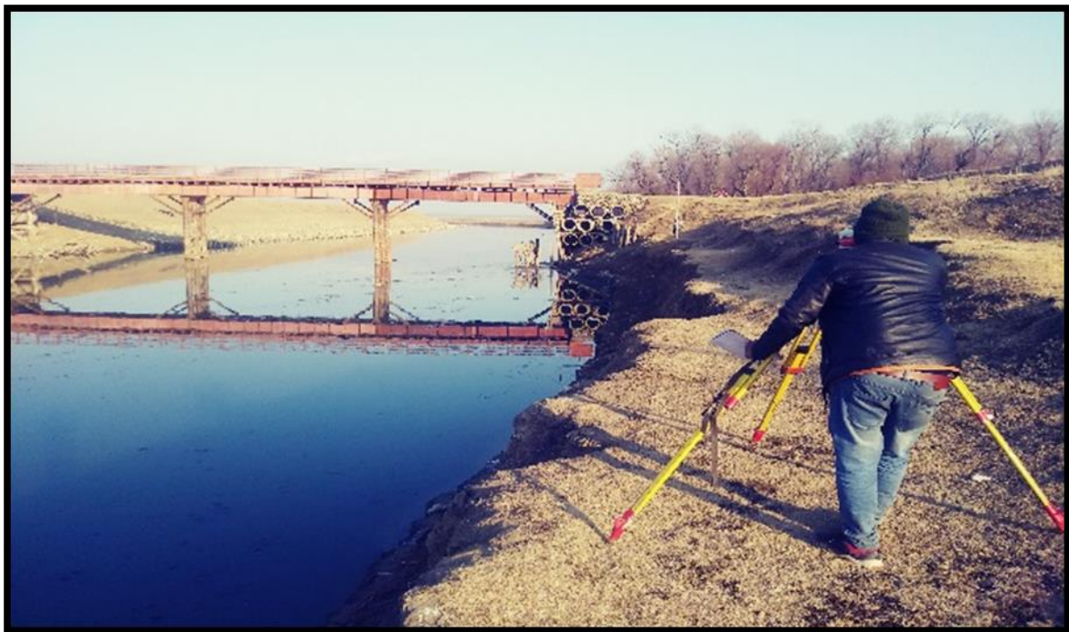
Figure 2.23 : CH- 44.20 Km Auto Level in Progress
