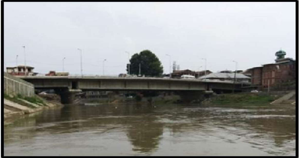
Figure 2.40 : Ch-117.73 Km Zene Kadal New Bridge
