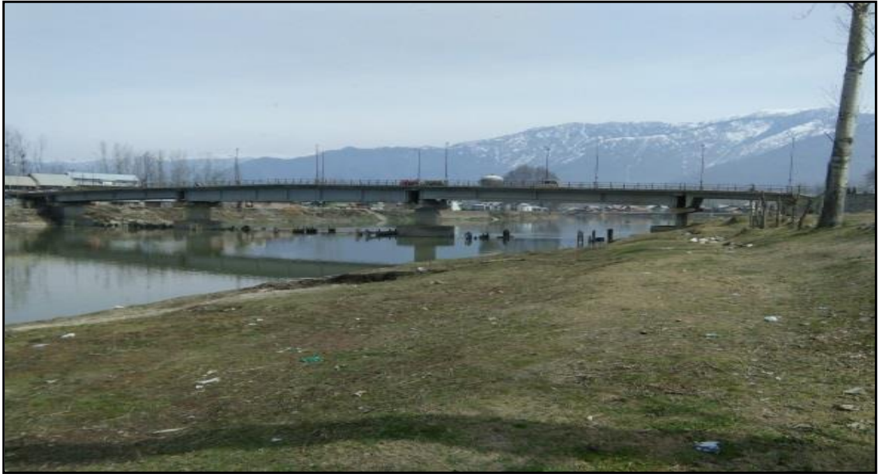
Figure 2.31 : Ch-79.95Km Hajin Bridge
