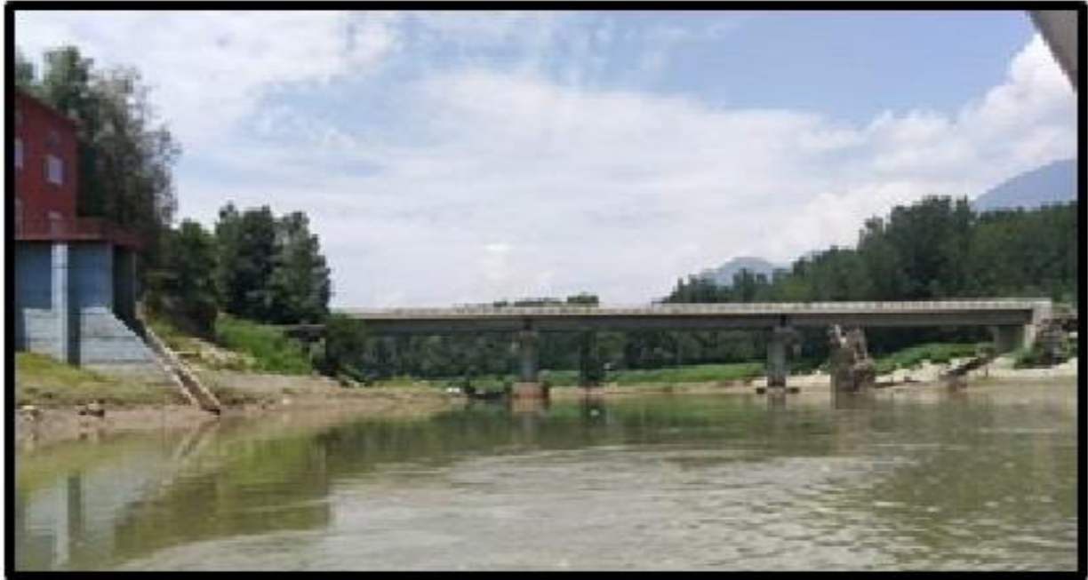
Figure 2.46 : Ch-165.63 Km Awanti Pura Bridge
