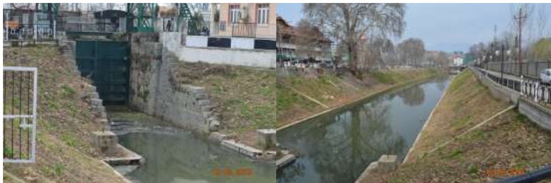
Figure 5-8 Canal connecting Dal Lake with Jhelum
