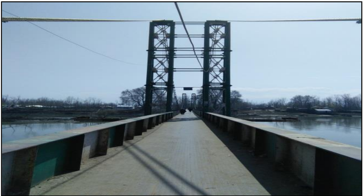
Figure 2.32 : Ch-87.94 Km Push Wari Bridge
