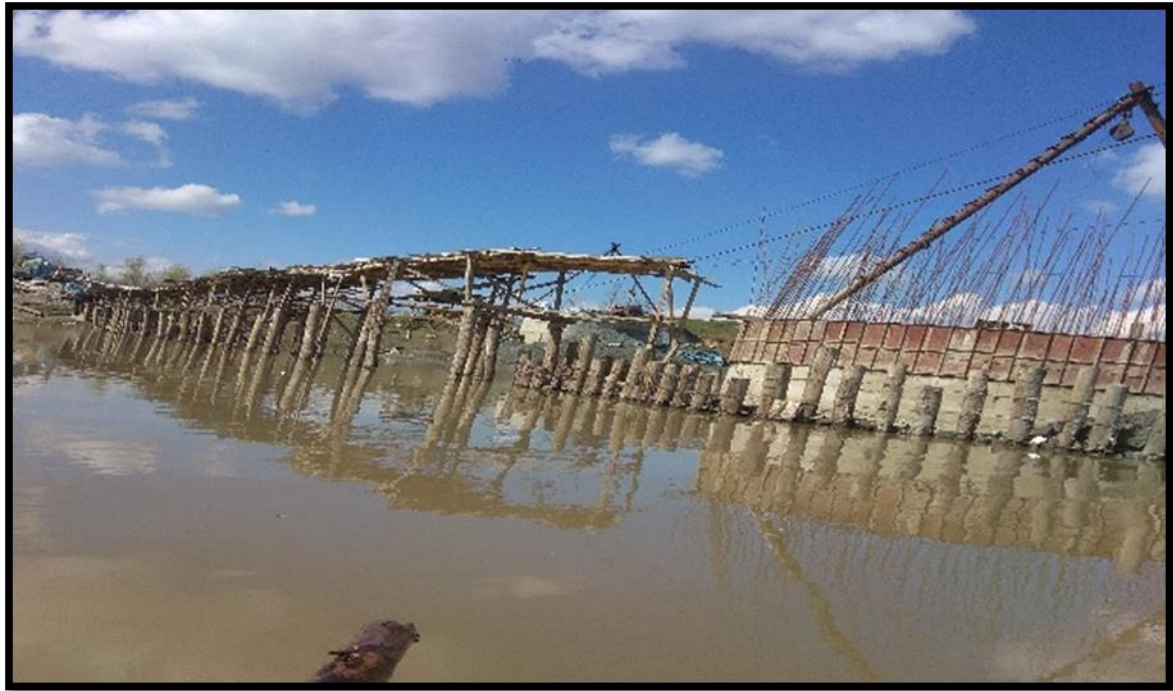
Figure 2.12 : CH- 36.50 Km Bridge Construction In Jhelum River
