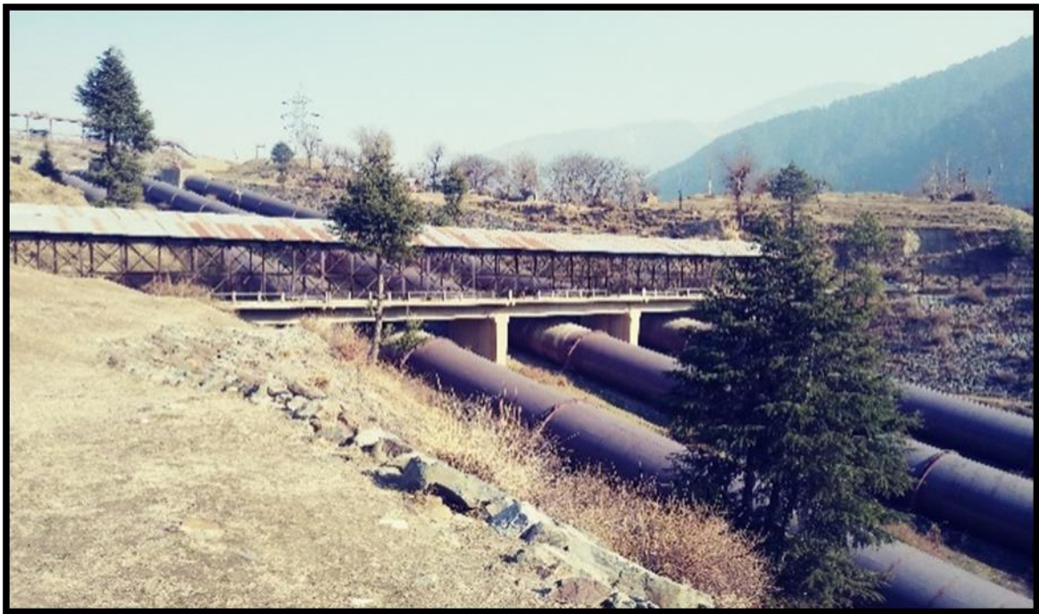
Figure 2.5 : CH- 0.40 km Water Supply For Turbine Through To Pipe Line to Generate Power
