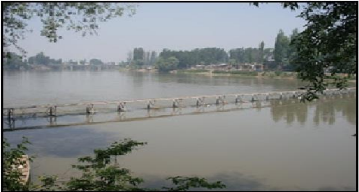
Figure 2.39: Ch-115.98 Km Chattabal Weir
