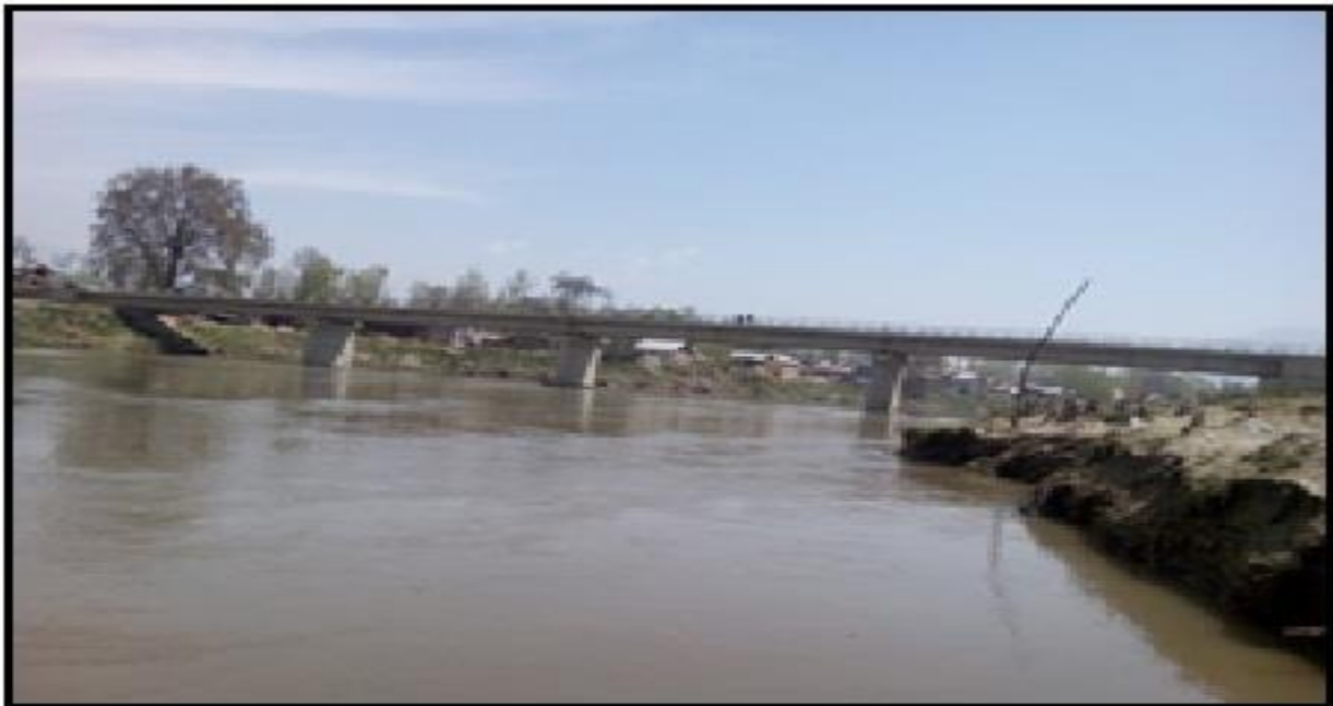
Figure 2.47 : Ch-171.00 Km Charsu Awantipora Bridge
