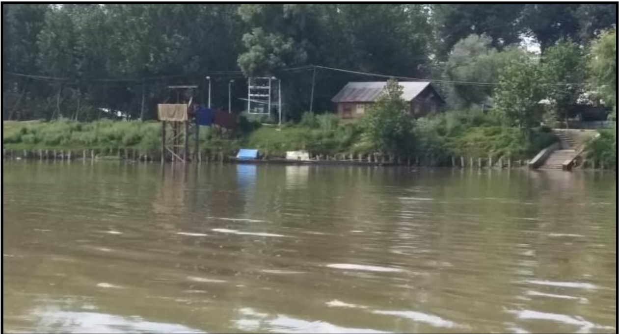
Figure 2.34 : Ch-99.33 Km Electric Line Crossing & Pump House
