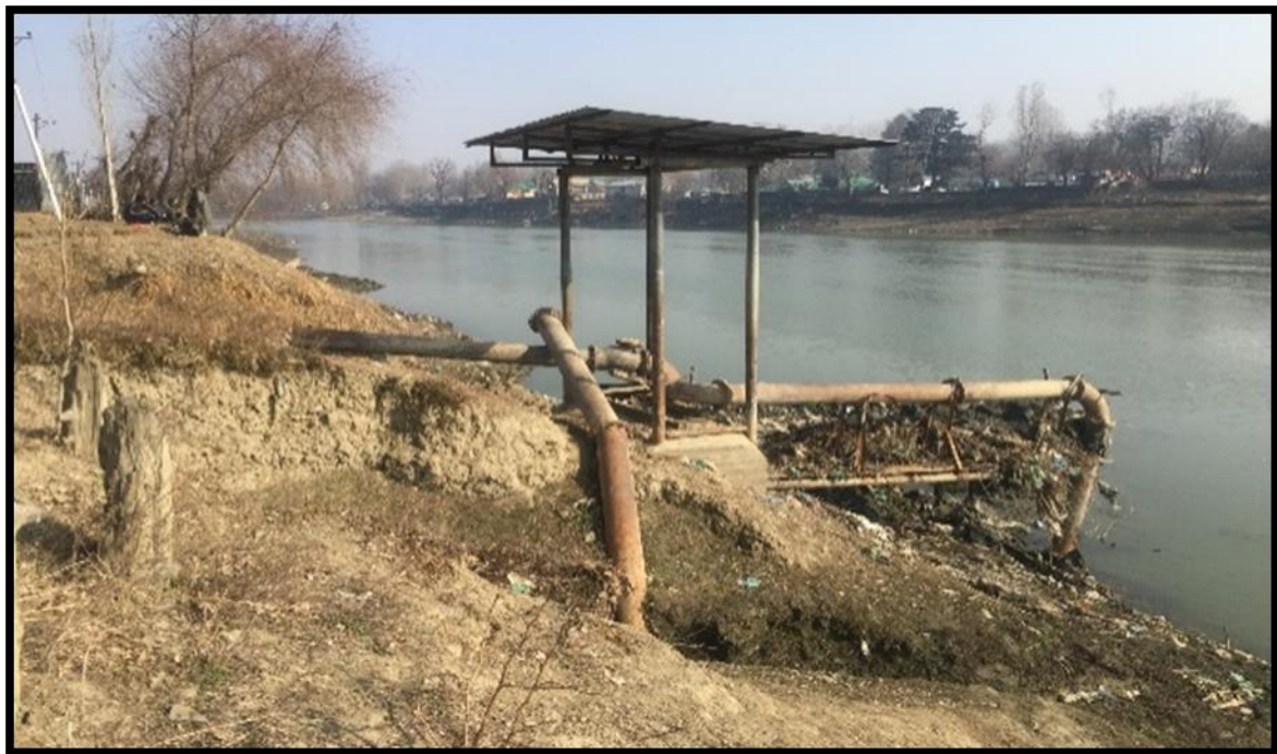
Figure 2.11 : CH- 22.81 Km View Of Jhelum River Pump House
