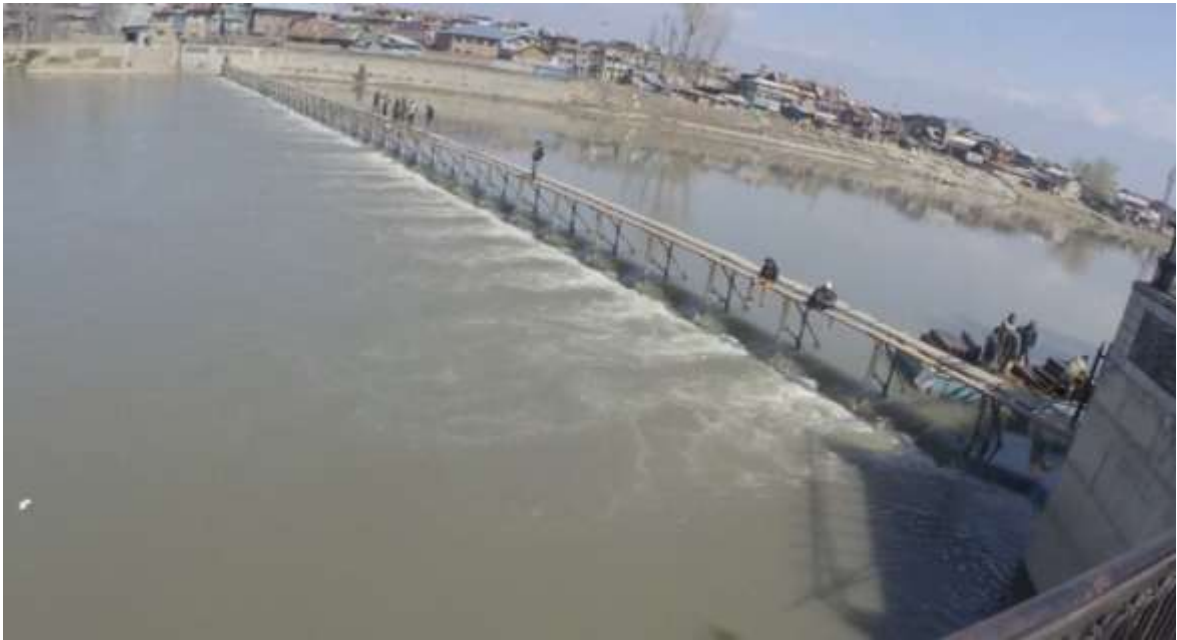
Figure 5-7 Chattabal Weir after removal of 9” blades
