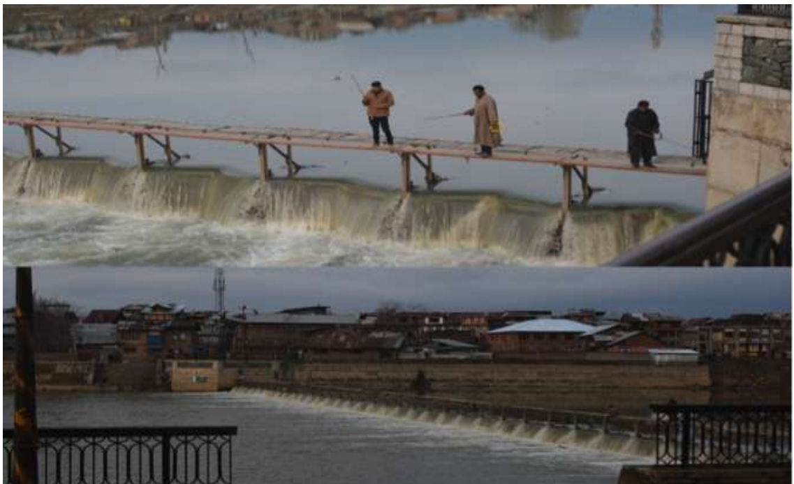
Figure 5-6 Chattabal Weir in Original Form
