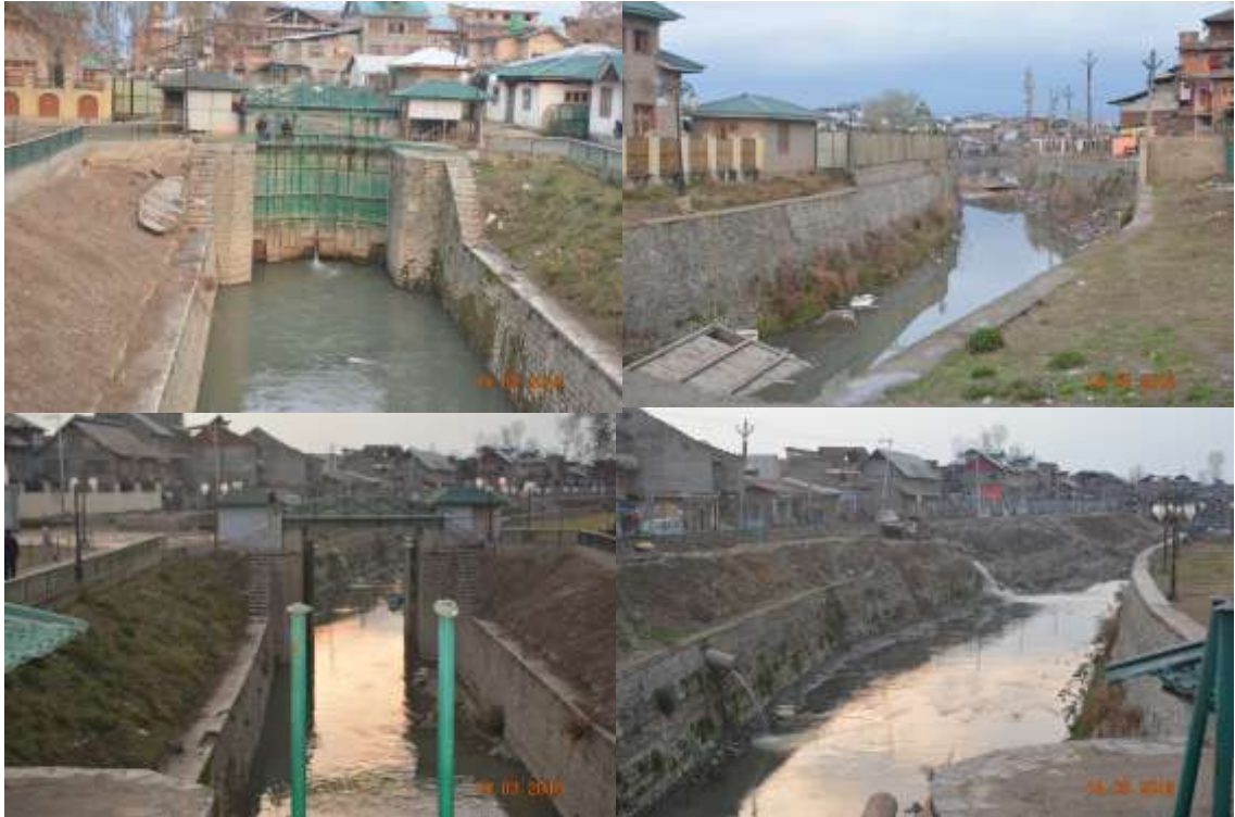
Figure 5-5 Lock Gates and Channel near Weir
