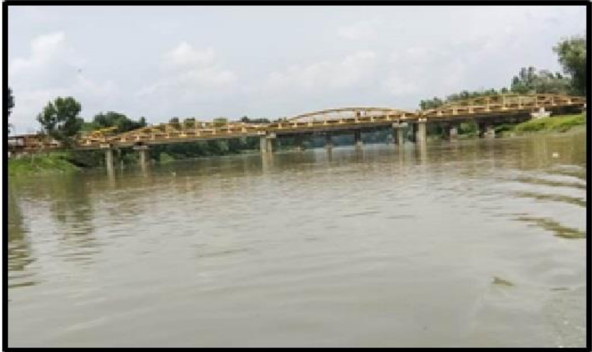
Figure 2.38 : Ch-111.03 Km Pipe Line Bridge Parimpura
