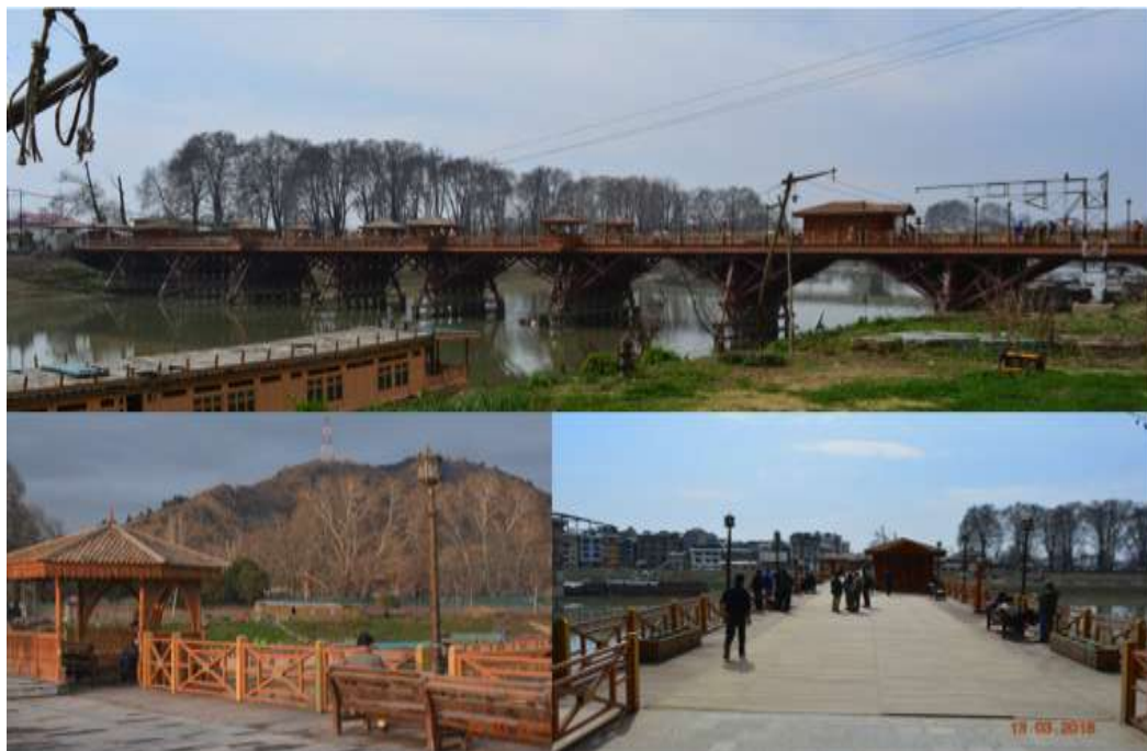
Figure 5-4 Zero Bridge on River Jhelum
