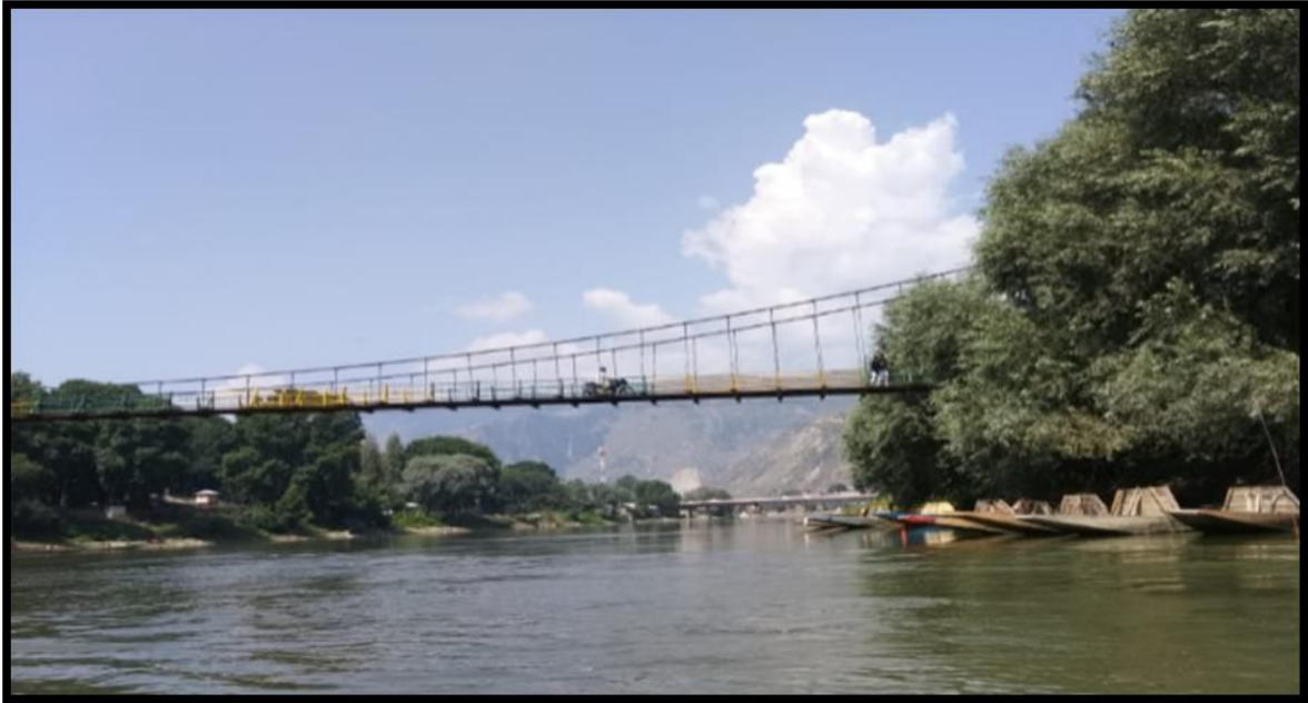
Figure 2.10 : CH- 19.94 Km Khanpora Bridge
