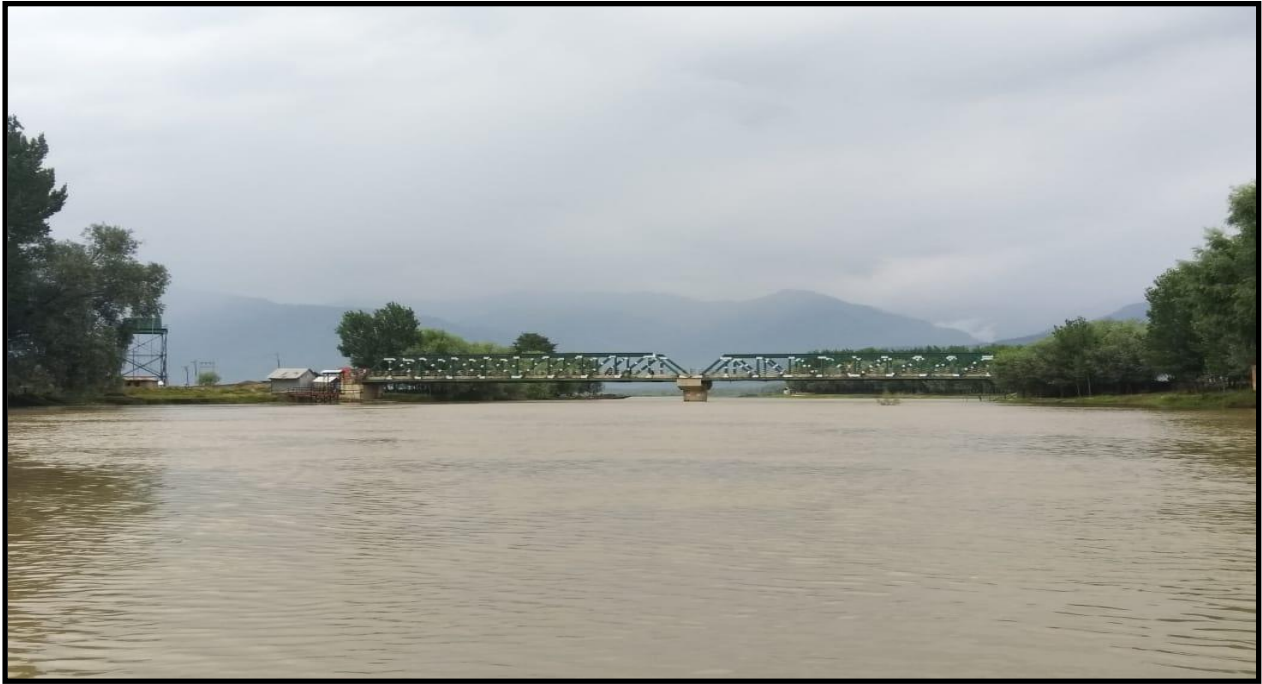
Figure 2.29 : Ch-73.73 Km Bridge & Pump House
