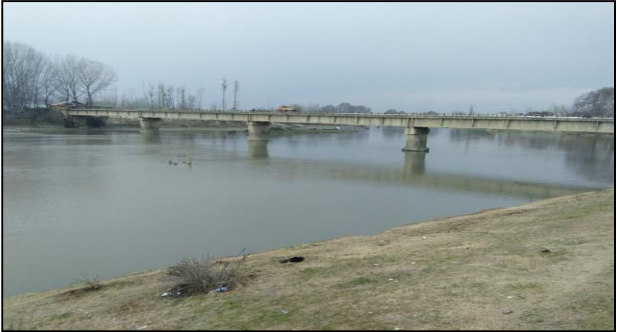
Figure 2.33 : Ch-91.01 Km Sumbal Bridge
