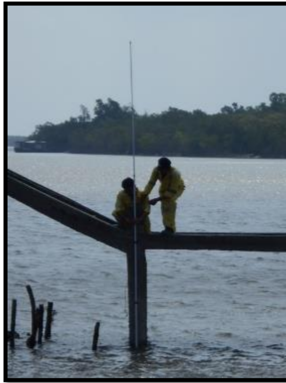
Figure 25: Tide Pole erection at Lothian
