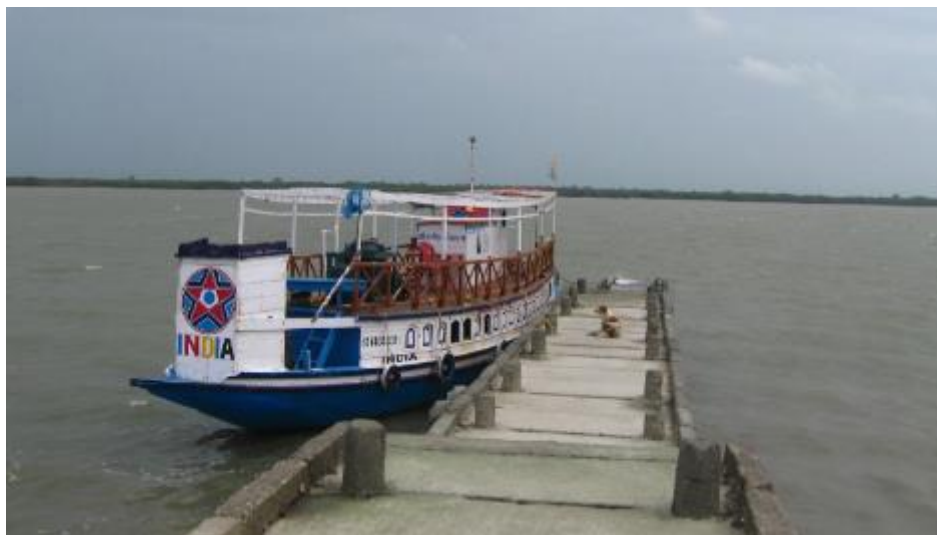
Figure 37: Facilities at Hemnagar Terminal
