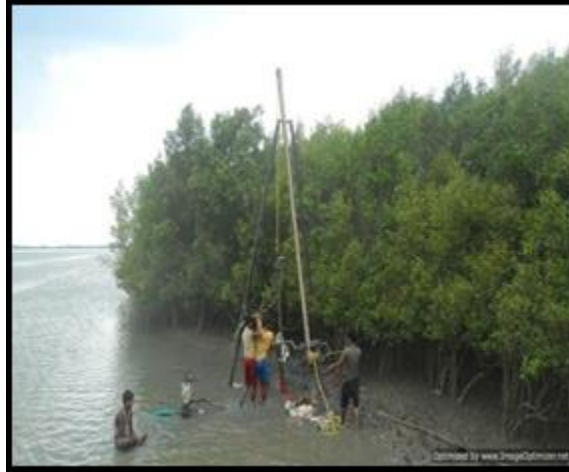
Figure 28: Erection of Tripod for Geotechnical Investigation
